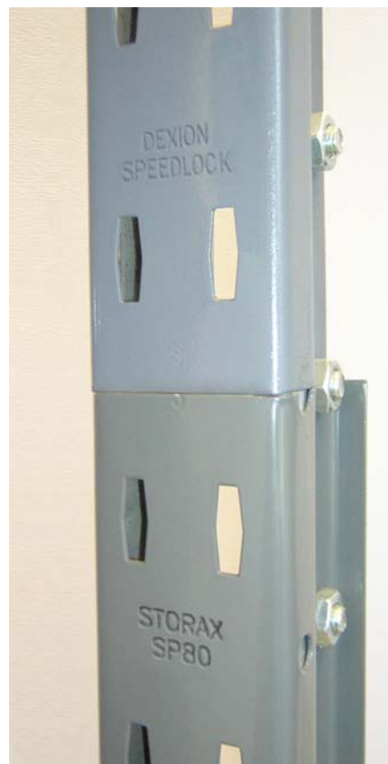
Original Dexion Speedlock® spliced with SP80
